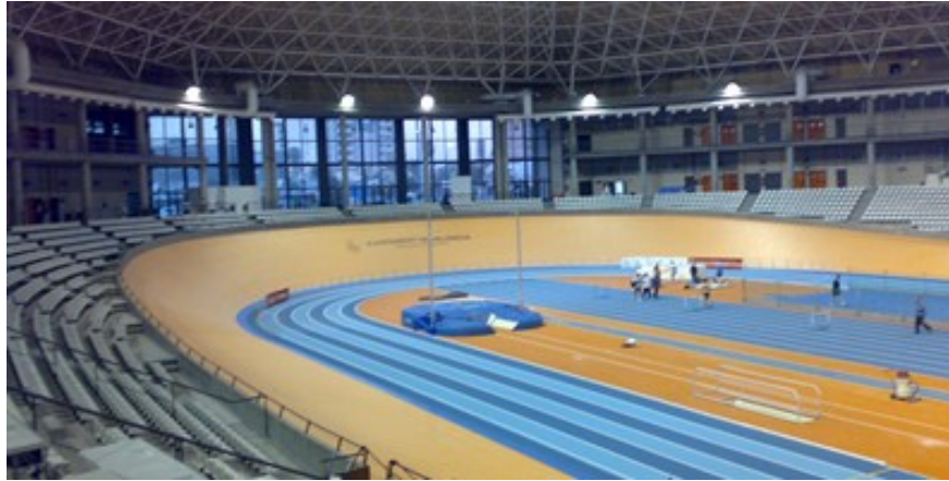
Figure 1. Interior of the velodrome [1]
