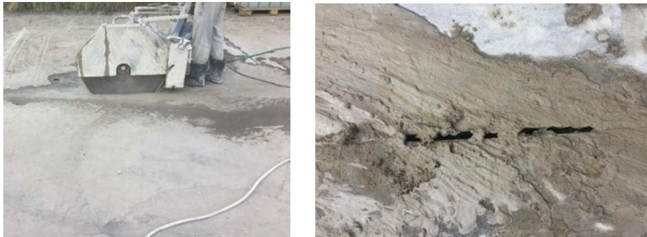
(A) The cutting process (B) A section of the injected plot after cutting
