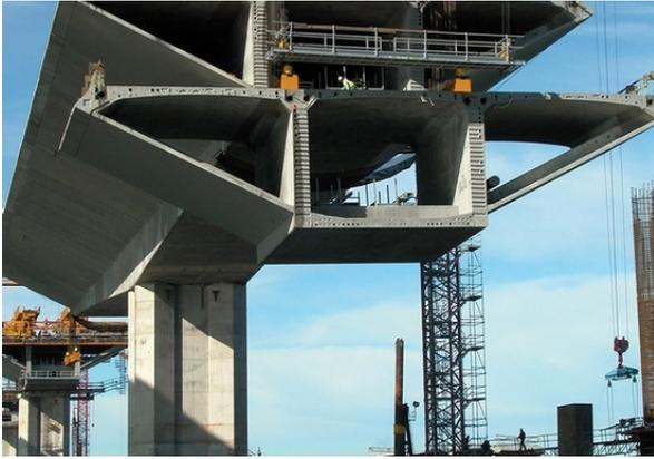
**Figure 1. Box-girder bridge multi-cell cross-section [23].**
