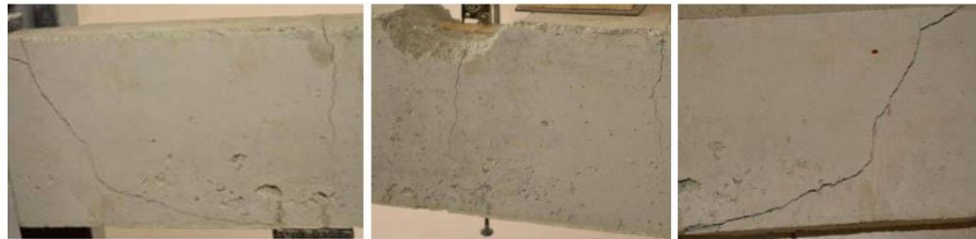
Figure 10. Cracking in the beam with fiber glass composite reinforcement.
