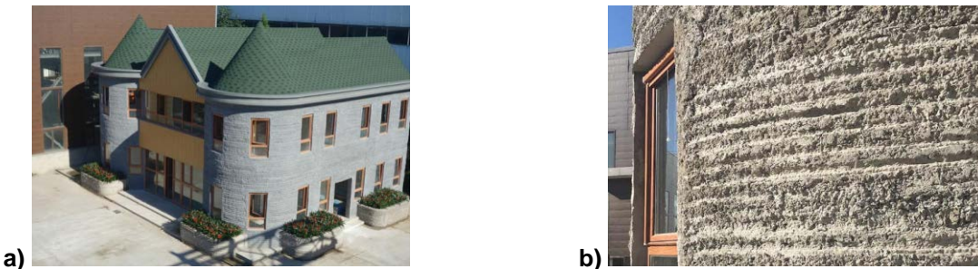
Figure 3. Typical 3D printing defects on the example of residential building by 'Tengda' (China) [12]: a), b) disruption of the geometrical dimensions due to spreading of the underlying layers, surface heterogeneity.
