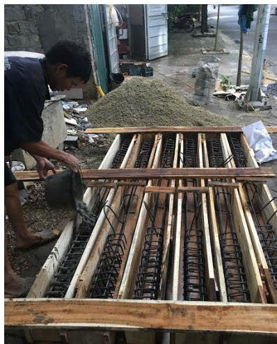
a) Formwork and reinforcement of beams
