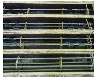
Wooden mold for casting beams
