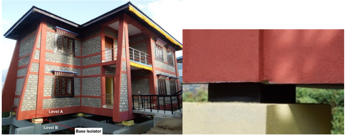
Figure 1. A view of the prototype base-isolated building [17].
