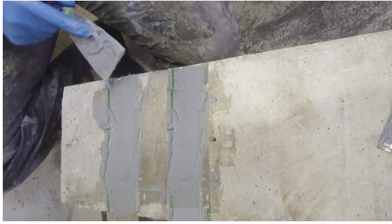
Applying the first layer of epoxy onto CFRP sheets surface
