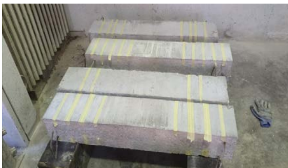
Marking the area of CFRP sheets bonded using plastering tape
