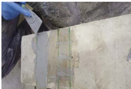
Applying the first layer of epoxy onto CFRP sheets surface
