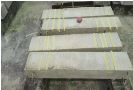
Marking the area of CFRP sheets bonded using plastering tape
