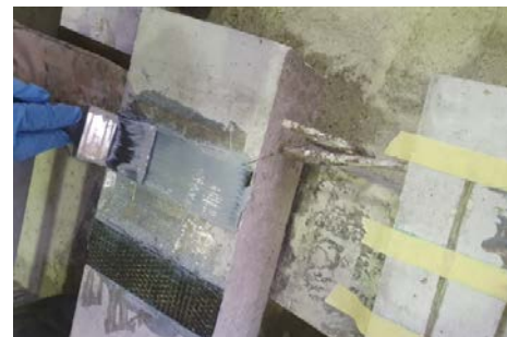
Applying the two layers of epoxy onto CFRP sheets surface
