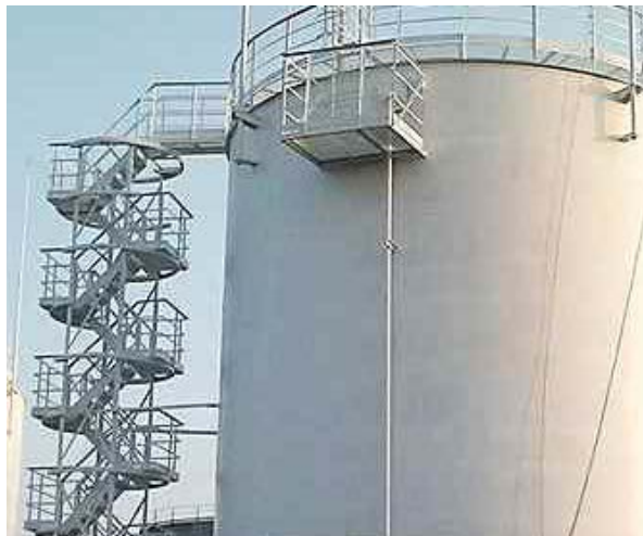
Figure 1a. Tank stair tower.
