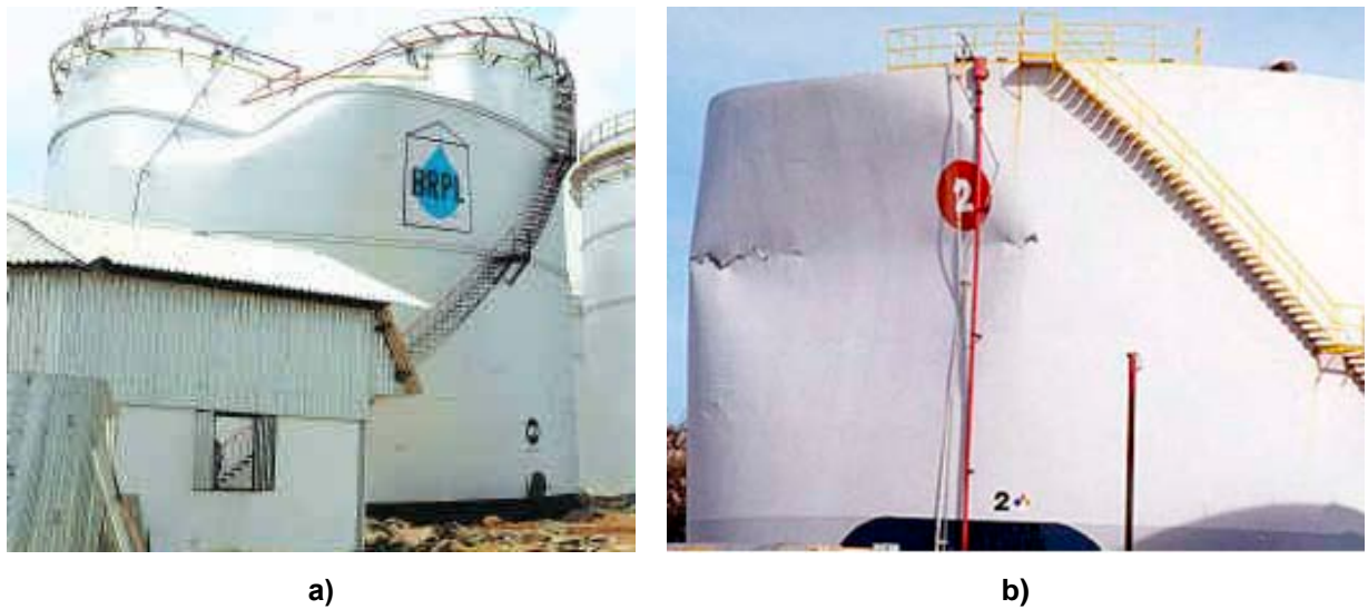
Figure 2. Buckling under the influence of wind.
