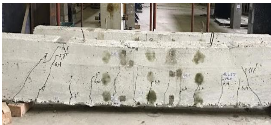
Figure 7. Formation and development of cracks in test beams.
