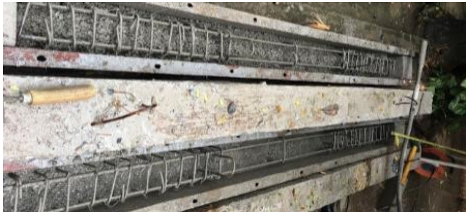
Figure 4. Concreting beams in layers.
