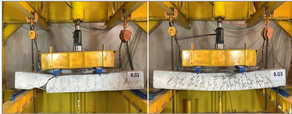
Figure 5. Crack pattern of the beams B.G1 and B.G3.
