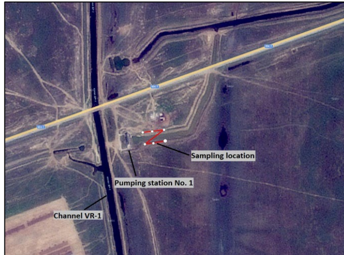
Figure 1. Places of concrete cores sampling.
