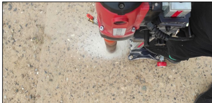
Figure 2. Process of cutting the cores using a diamond drilling rig.
