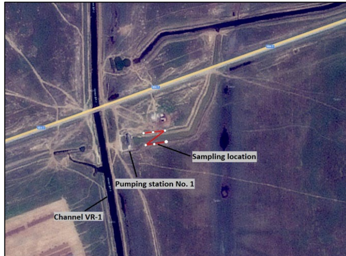
Figure 1. Places of concrete cores sampling.
