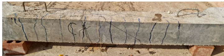
(a) Crack pattern for 450 °C temp. Specimen.
