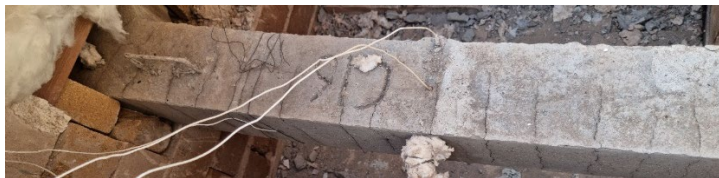
(b) Crack pattern for 600 °C temp. Specimen.
