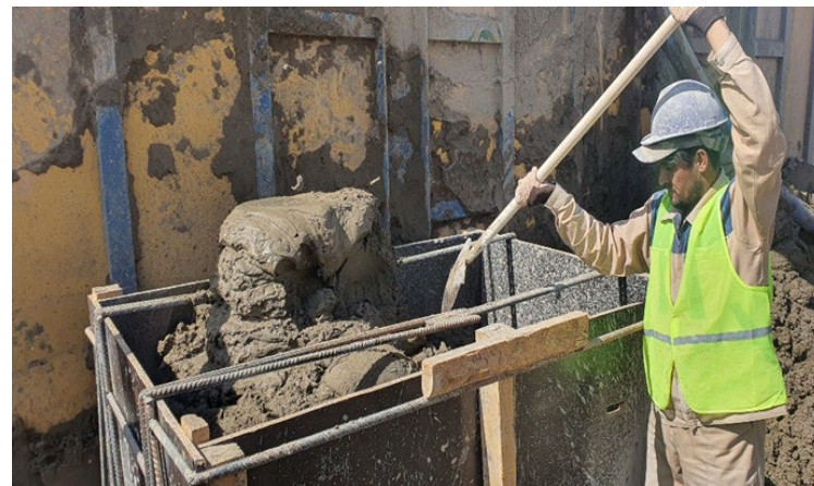
Figure 5. Collect sludge and sand in-container.
