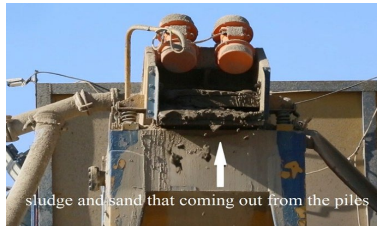
Figure 4. Filter sand and sludge by desander in-situ.
