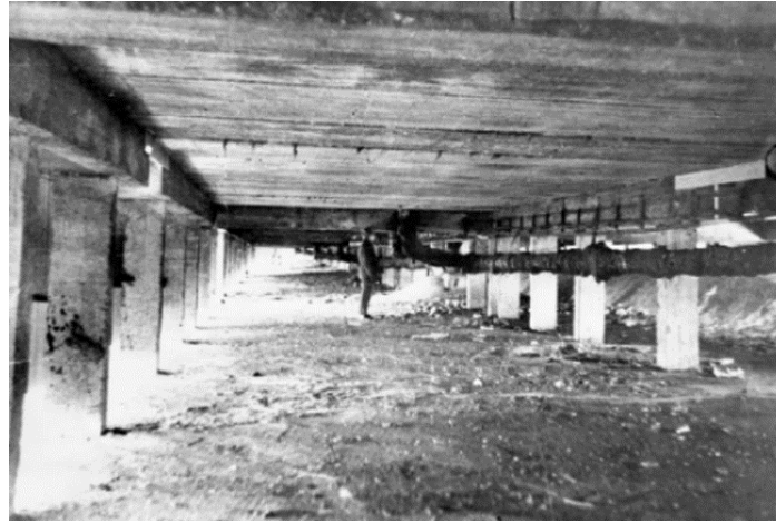
Figure 1. Ventilated underground space of a residential building on permafrost soil.
